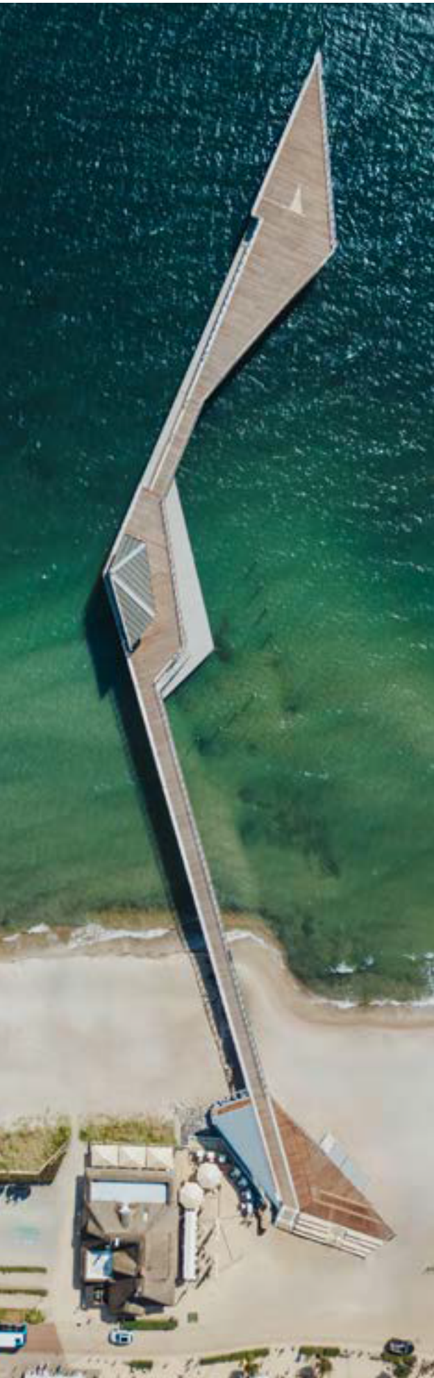
The pier shortly before opening Image on the left and images below: © TALB / Joelle Dörnath
