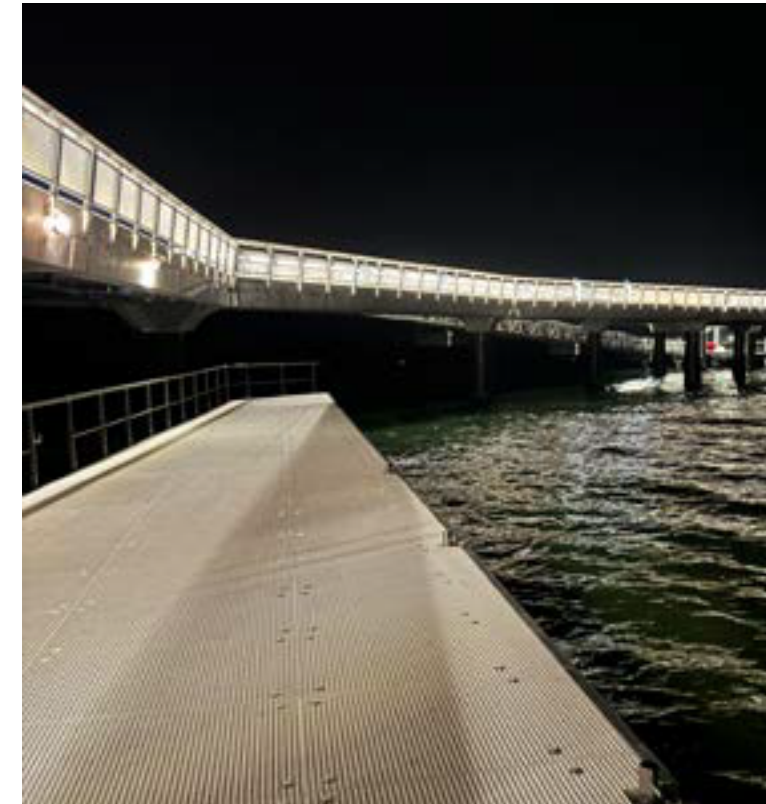
The illuminated pier construction. © CHRISTMANN + PFEIFER
