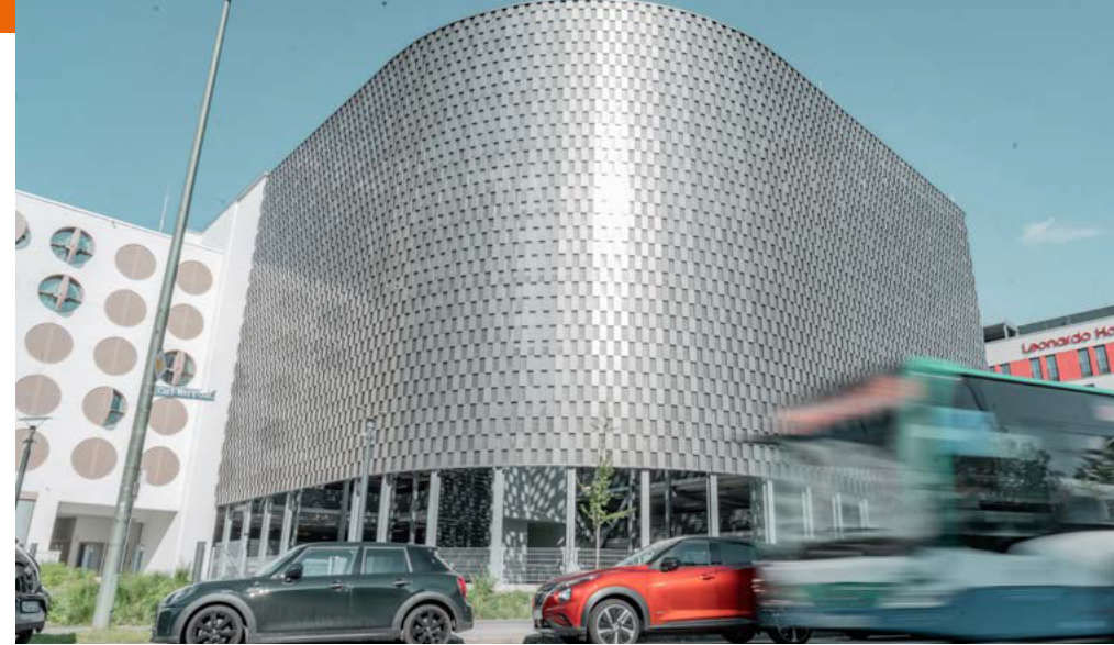
17,000 facade tiles cover the 24-meter-high building on Carl-Wery-Straße.
