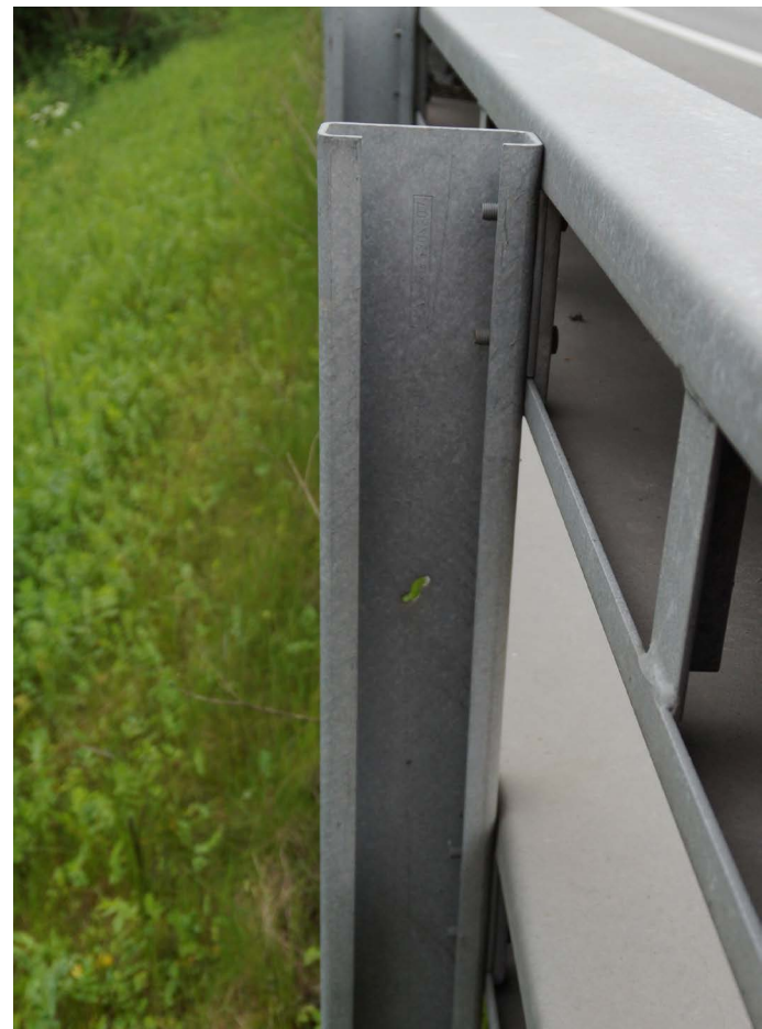
Fig. 2: Thin-film "microZINQ®"-galvanized C-profile posts after 10 years.
