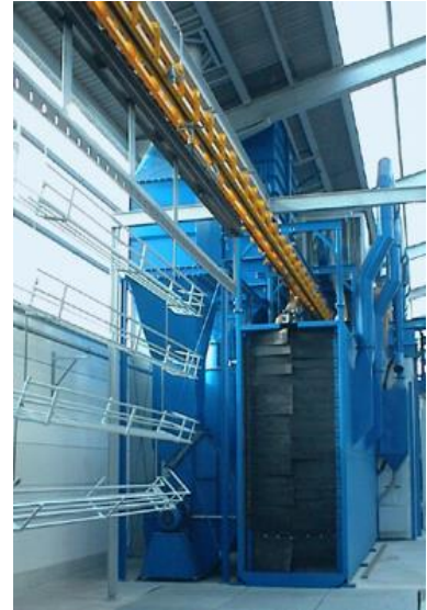
Installation de grenailage
